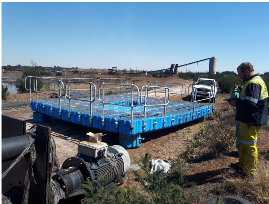
The MRS installed pump floatation device ready to be fitted with a vertical spindle pump
